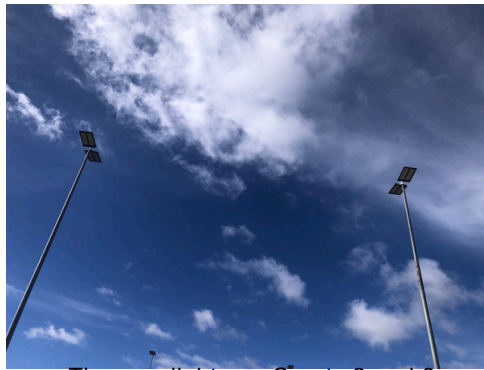
The new lights on Courts 2 and 3
