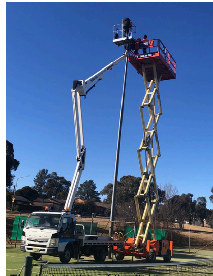
The installation of the lights on Courts 2 and 3
